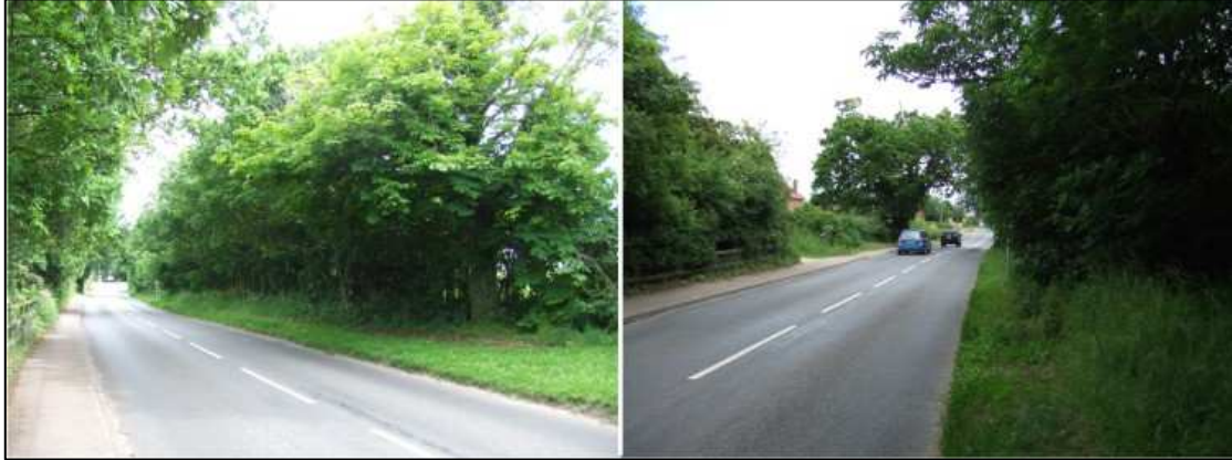
Figure 3.5: Creating an access at Point A would require the removal of mature trees (shown in photo on left) to create the required visibility splay. Also, the slight curve in the road exacerbates the land take required
