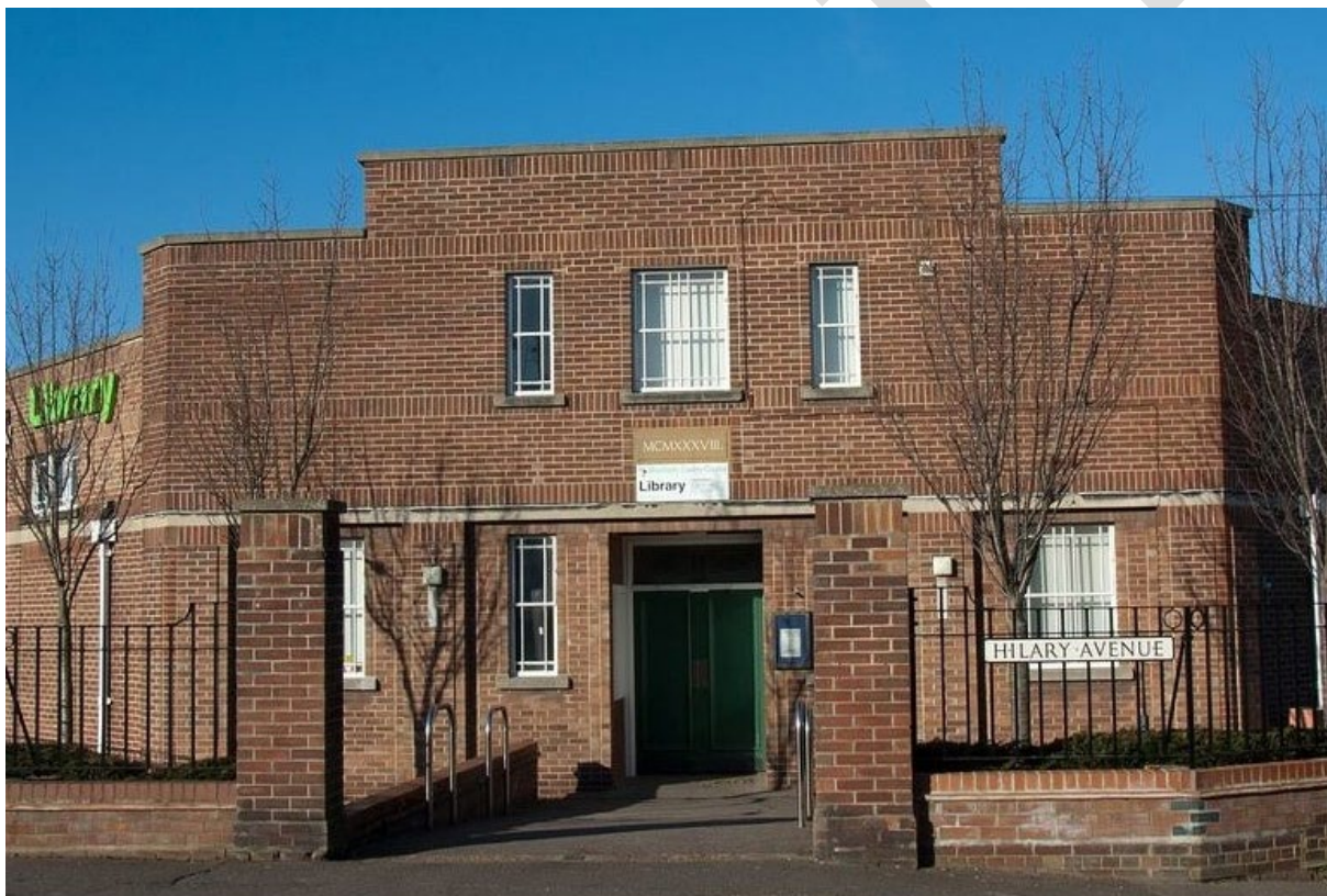
Figure 3 - Plumstead Road Library
